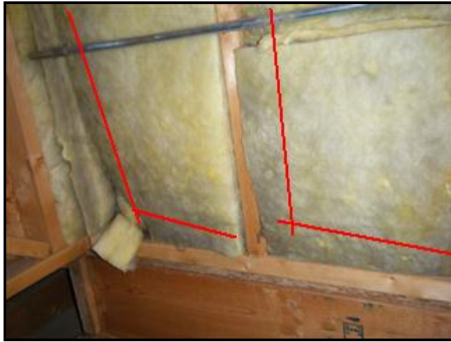
9.6 Picture 1 Fiber glass filtering air flowing in toward the wall
