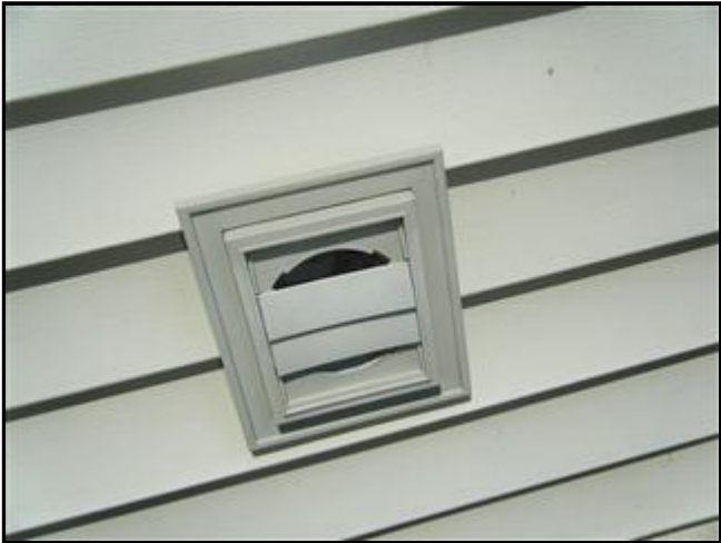
9.4 Picture 1 Vent flaps missing
