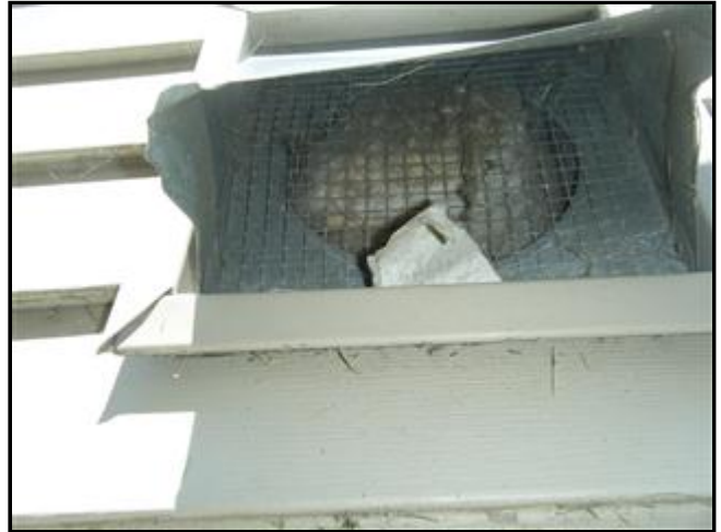
9.4 Picture 3 Intake vent packed with insulation
